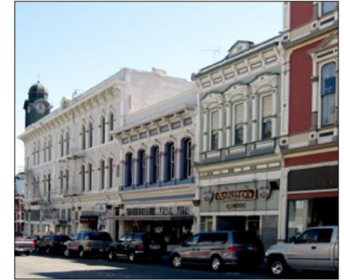
Illustrative Photo: Commercial blocks with retail uses on ground floor
